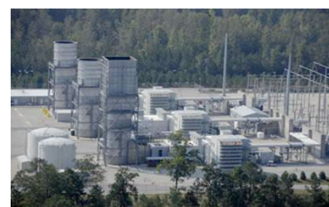
Hawk Road Energy Facility
