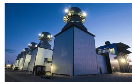
Talbot Energy Facility
