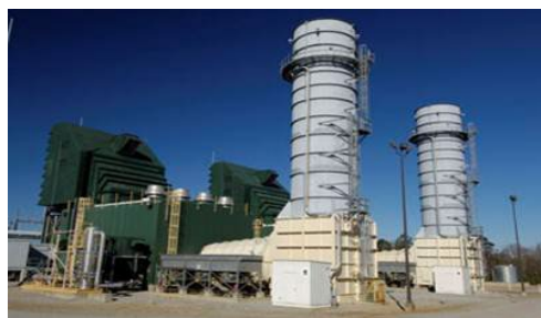
Smarr Energy Facility
