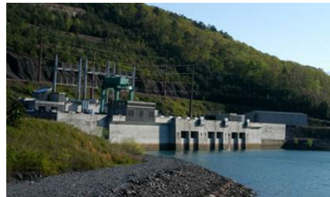
Rocky Mountain Hydroelectric Plant
